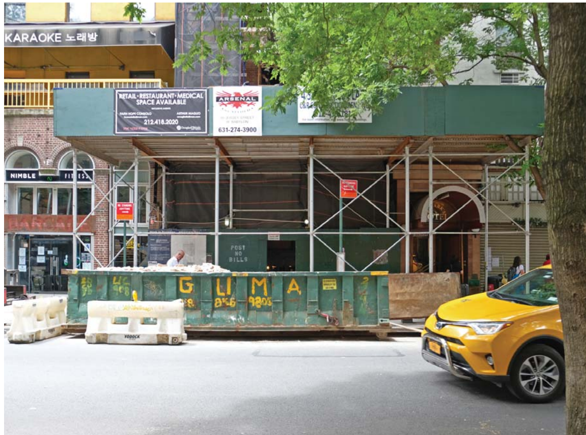
3. VIEW ACROSS ST. MARKS PLACE LOOKING SOUTH TOWARD LANDMARK SITE Photograph Taken June 20, 2018
